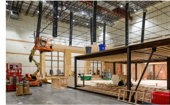
Construction of a sound stage within a movie studio
