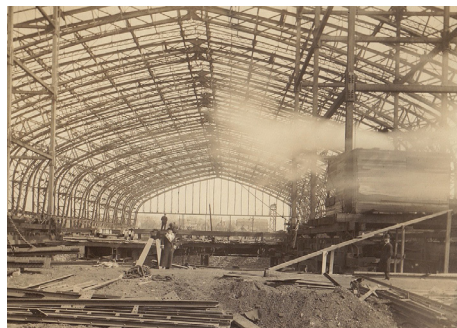
Drill hall during the construction of the Kingsbridge Armory
